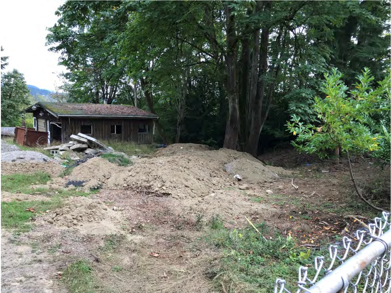
Exhibit 1-C: Stop work order removed; Additional grading. Photo taken 10/09/2020.
