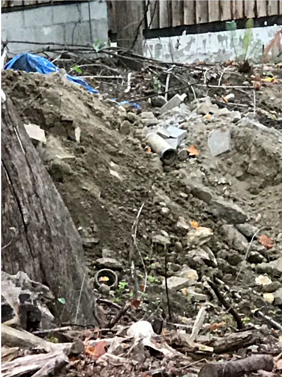
Exhibit 3-B: Debris in soils Photo taken 10/07/2020.
