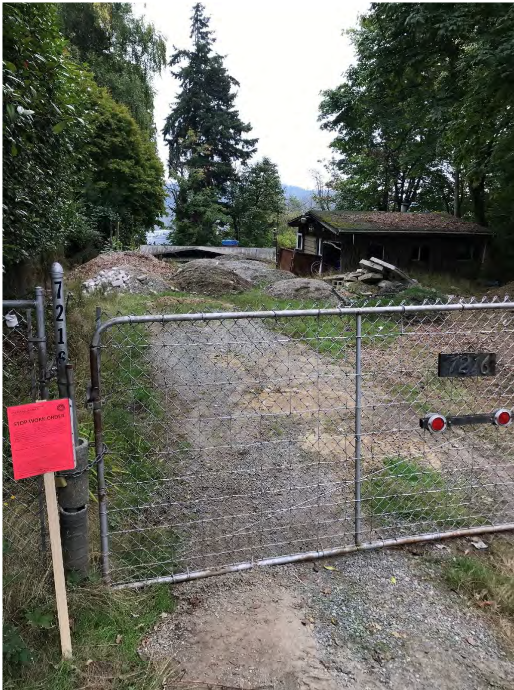
Exhibit 1-B: Condition of site at time of SWO Photo taken 10/07/2020.
