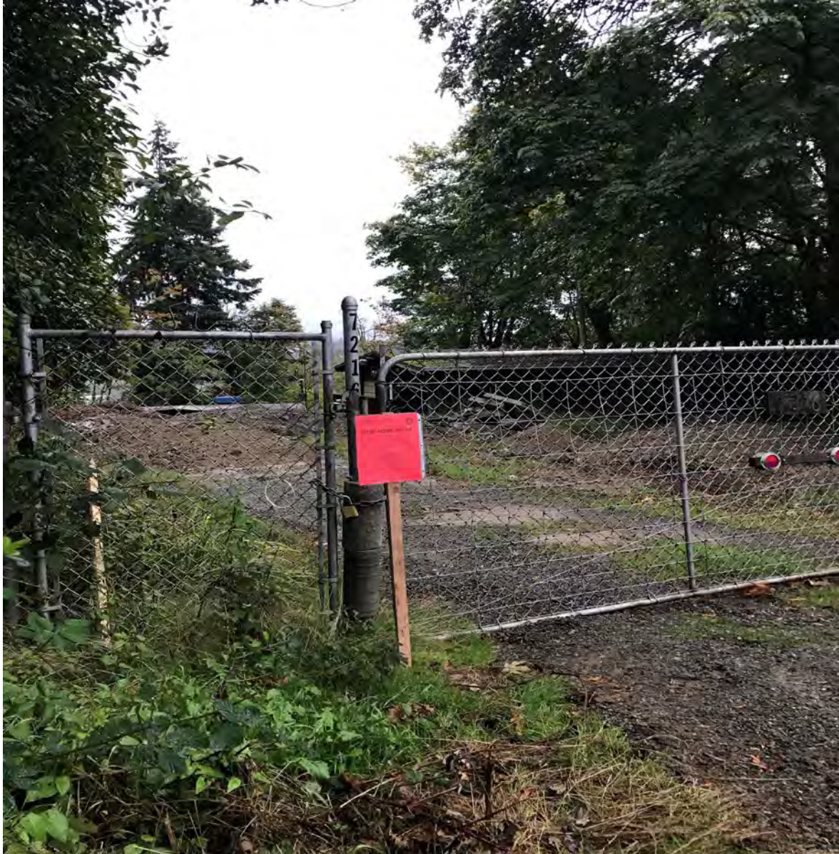
Exhibit 1-D: Second Stop Work Order Posted Photo taken 10/19/2020.
